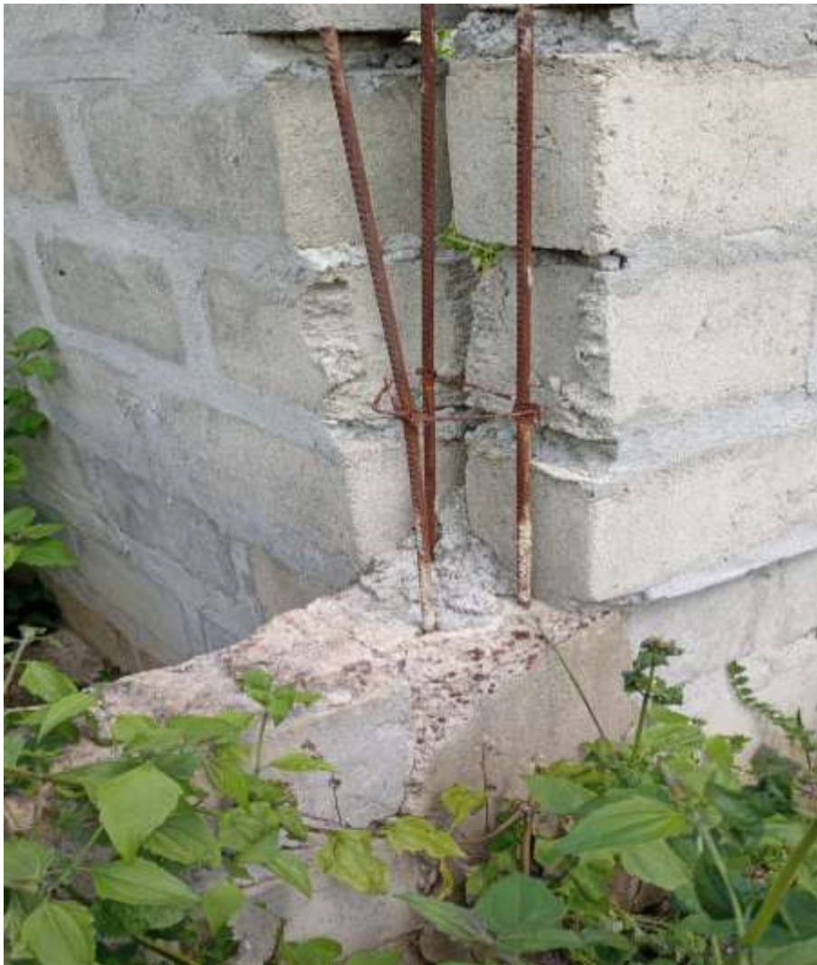
Figure 31.0 Elementary School Construction: Substandard Rocks
