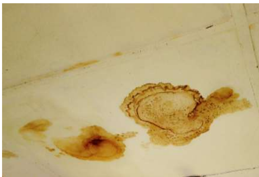
Figure 23.0 Leakage in Commissioner compound (Substandard)
