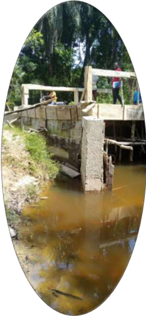
Figure 3.0 Gbarlorkpalah Bridge Project: Wingwall placed far from the water bank (Substandard Work)
