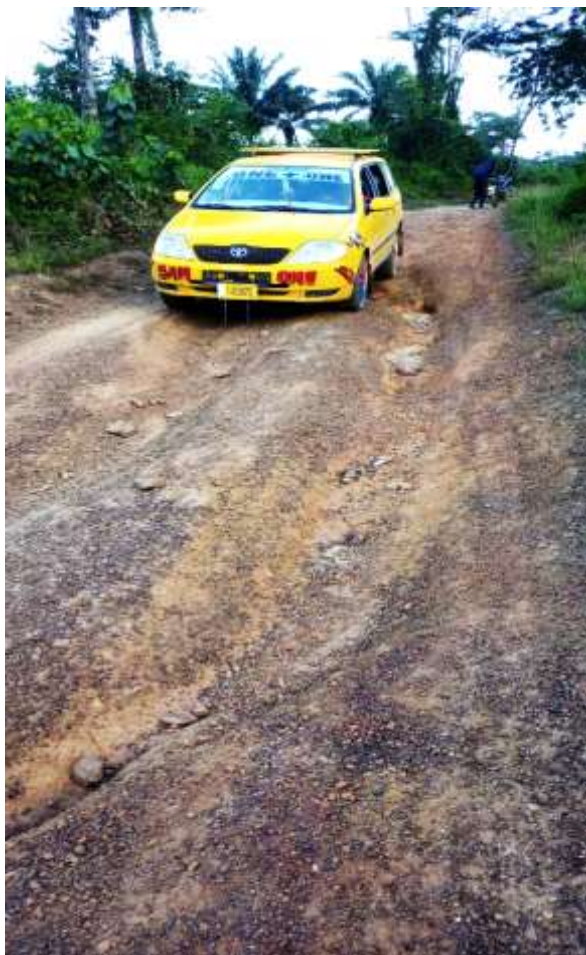
Figure 11.0 Rehabilitation of 6.8 Kilometers road: (Substandard work)
